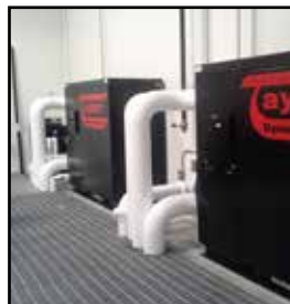
Coolant Storage and Distribution
